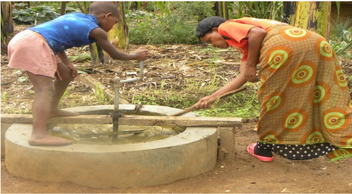
Figure 5: Showing household members in Greater Bushenyi using a locally fabricated dung mixer to replenish their biodigester
