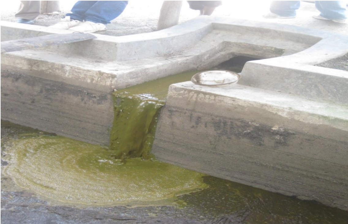
Figure 6: Showing the recommended viscosity of bioslurry, flowing into the slurry pit
