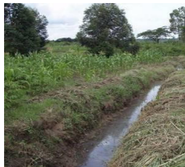
Cleared drainage by community members
